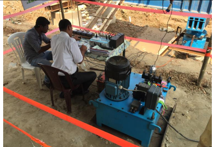
Supervision and recoding of load test data from a safe distance.
