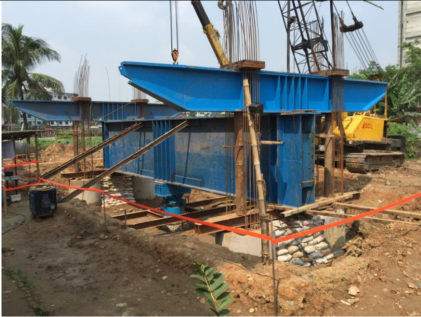
Load Test Arrangement. Test Frame weighing 40T manufactured at DCL yard. Test Pile 1200mm diameter 60m length constructed by DCL.
