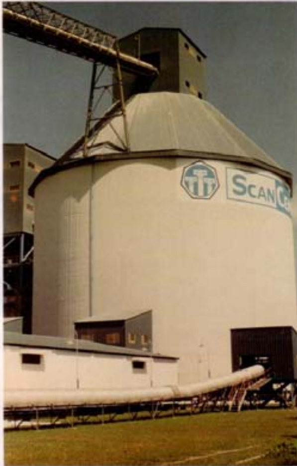
36m diameter and height 32m, Capacity 40,000 Ton Clinker Silo using SLIP FORM Technique
