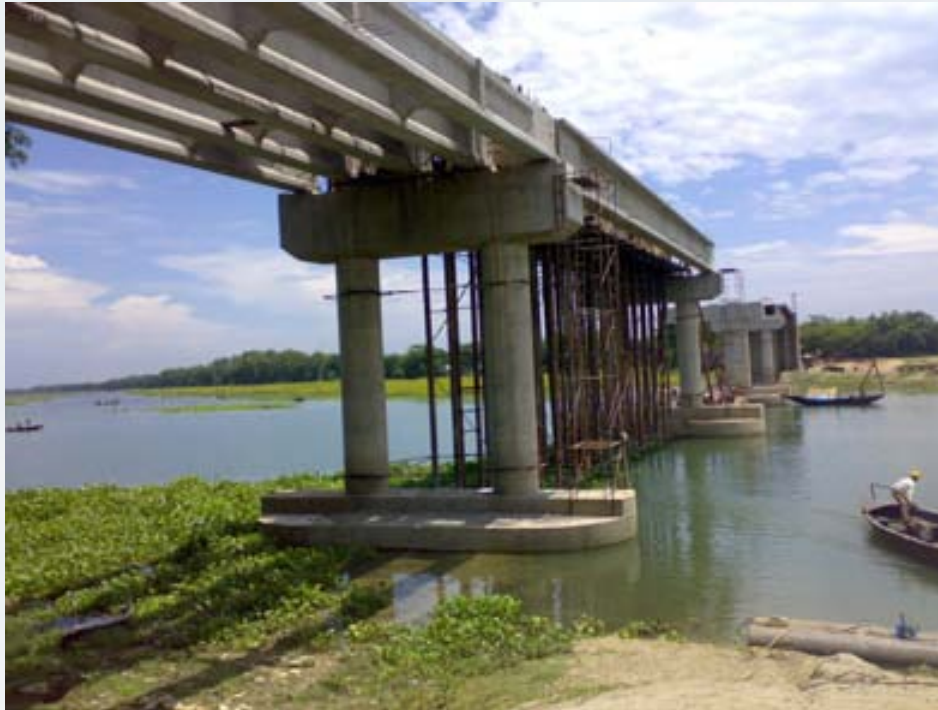
Construction of 38m long Pre-stressed Girder
