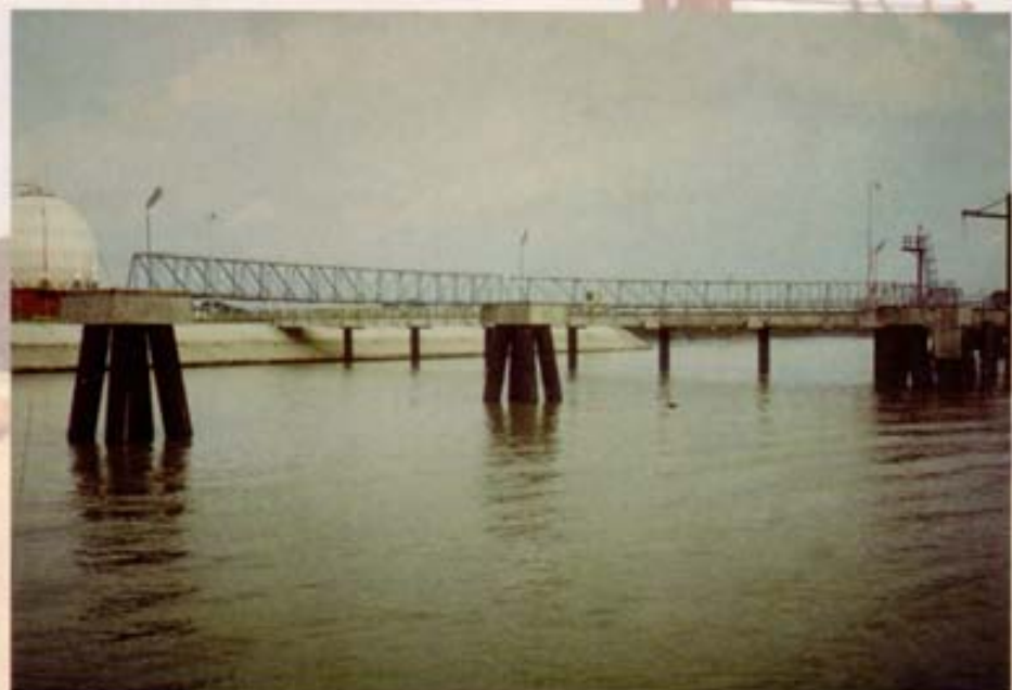
Completed Dolphin Jetty for 3800 DWT, LPG Vessel Berthing
