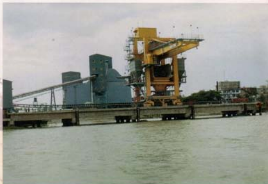
Completed Jetty 73m x 14m with 8m x 72m catwalk with 120 Ton capacity Gantry Crane for Dhaka Grinding Plant Project of SCANCEN
