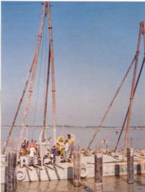
Off-shore Rotary Drilling for Bored Cast in Situ R.C.C. Pile for Jetty, Meghna River.
