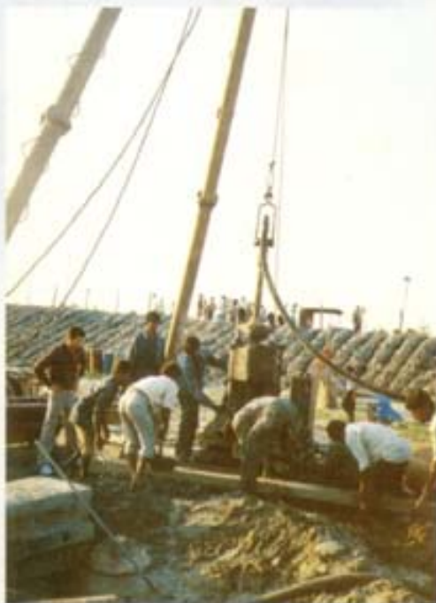
Construction of 1.2 metres Dia and 36 metres Long Cast-in-Situ R.C.C. Piles by Rotary Drilling Method at Str. No.-20, Contract No-9, RIP Project, Faridpur.
