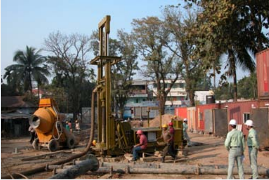
Reverse Circulation Drilling
