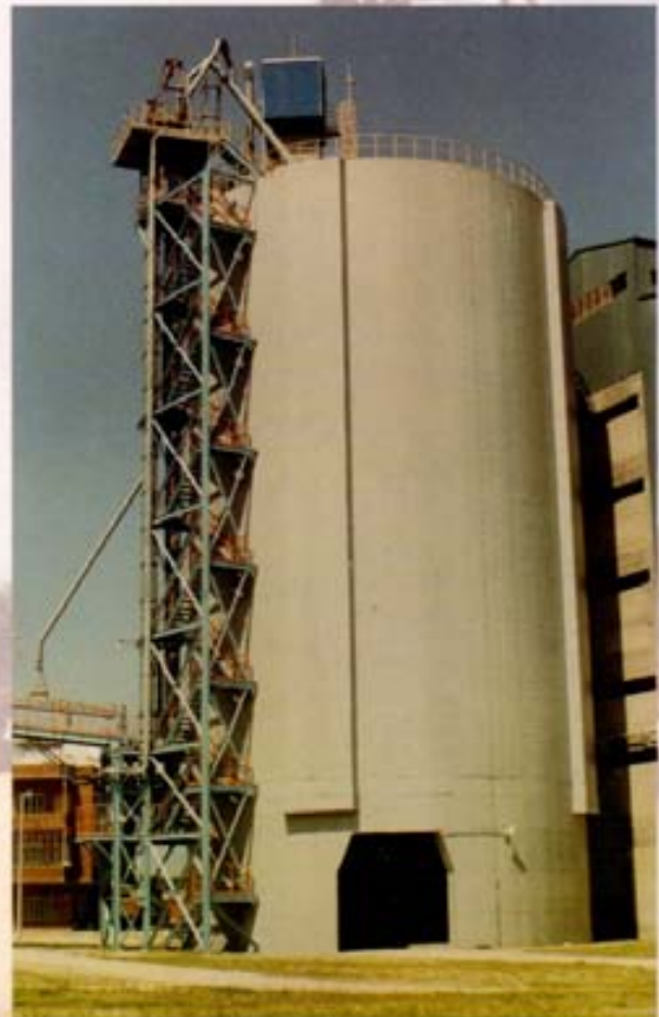
16m diameter and height 33m, Capacity 5,000 Ton Cement Silo with Pre-stressed Concrete shell using Slip Form Technique
