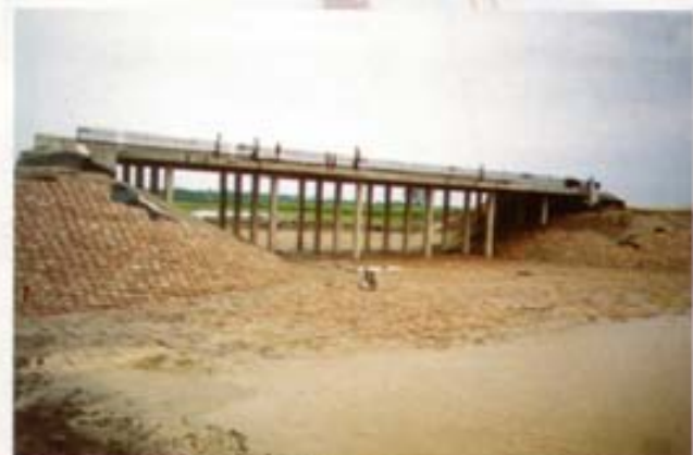
Slab Bridge (31 m) on 28.4 m Pre-cast Driven Pile at Ch : 1+475, Contract No. 3, JMB Project, Tangail
