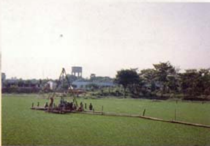
Soil Investigation Work by Tone Boring Rotary Rig for the proposed Water Garden Hotel, Dhaka, Bangladesh
