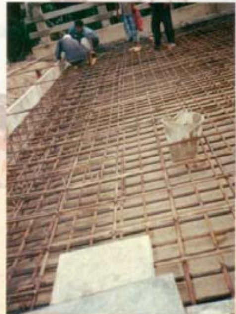
Re-bar Placing for Approach Slab at Str: 46, Contract No. 11, RIP: Jhenaidah
