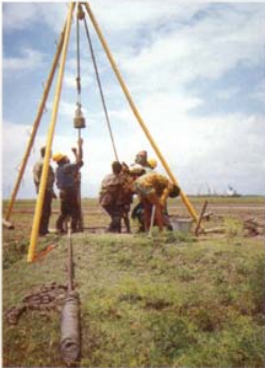
Environmental Assessment, Drilling with 150mm diameter Auger, collection of soil & water and installation of Monitoring Wells.
