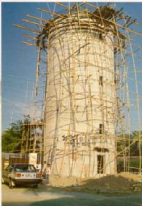
Construction of Vertical Shaft
