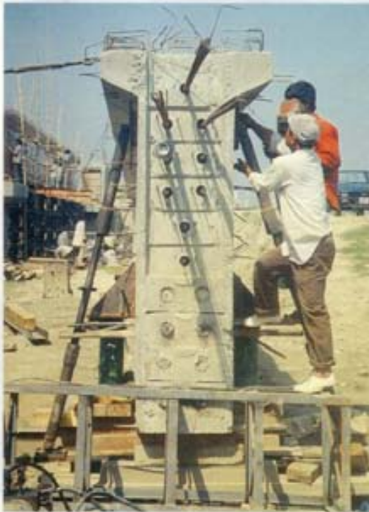
Arrangement for Pre-Stressing the Cables (Final Stage) at Str: 46, Contract No. 11, RIP Project, Jhenaidah
