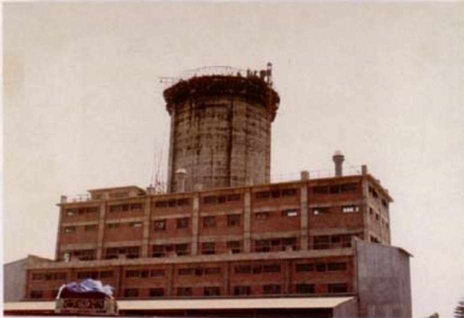
Completed Packing Building and under Construction 5000T Cement SILO using Slip Form
