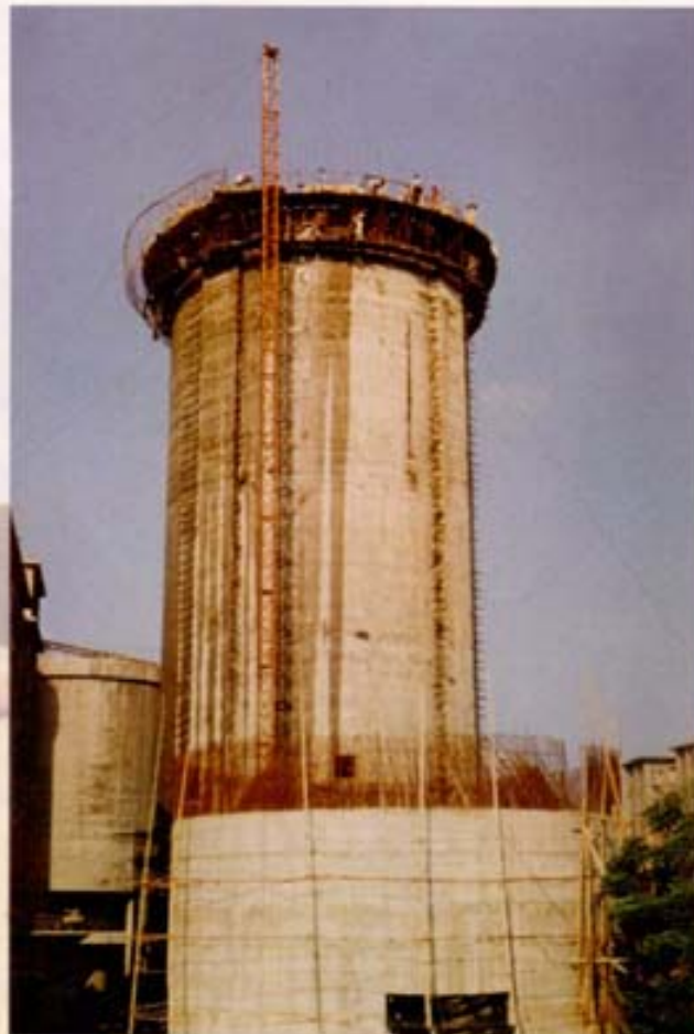
Completed Cement SILO by SLIP FORM
