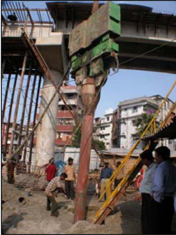
Ground improvement using vibro-compaction for reinforced earth ramp at Malibagh
