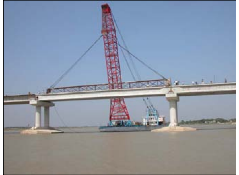
Erection of PSC Girders on bridge piers
