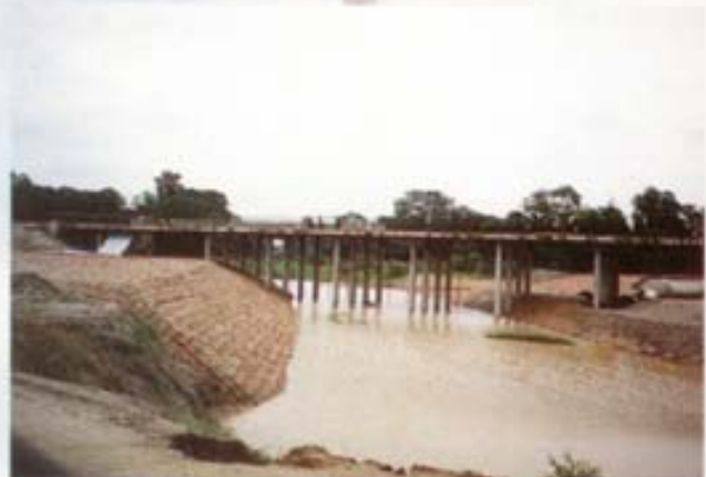
Slab Bridge (66 m) on 28.4 m Pre-cast Driven Pile at Ch : 6+818, Contract No. 4, JMB Project, Serajgonj
