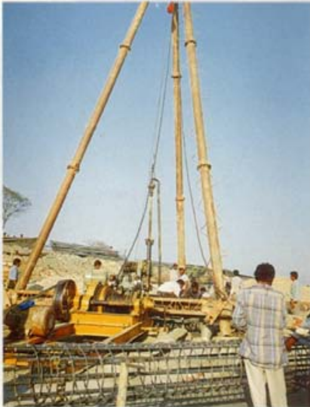
Construction of 600 mm Dia and 45 m long Cast-in-Situ R.C.C. Piles
