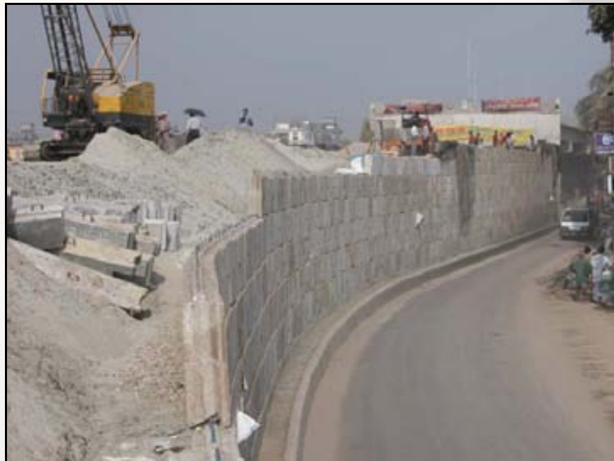
Segmental retaining wall at Saidabad ramp
