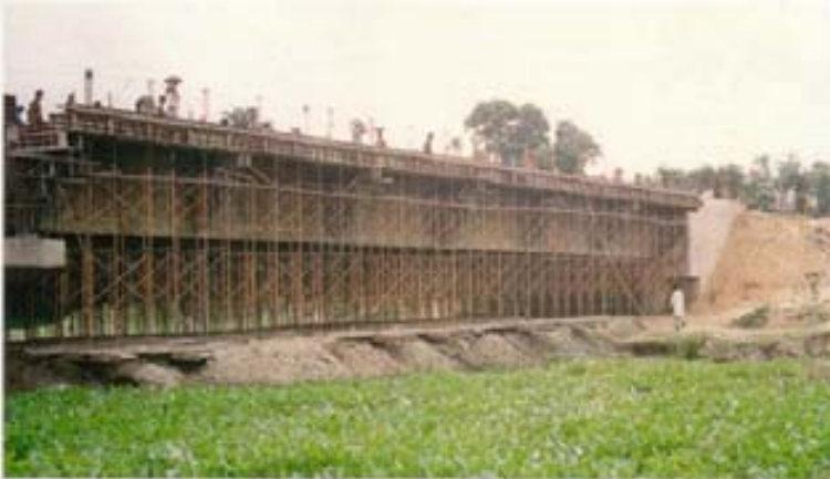
Preparation for Deck Slab Construction at Str: 46, Contract No. 11, RIP: Jhenaidah
