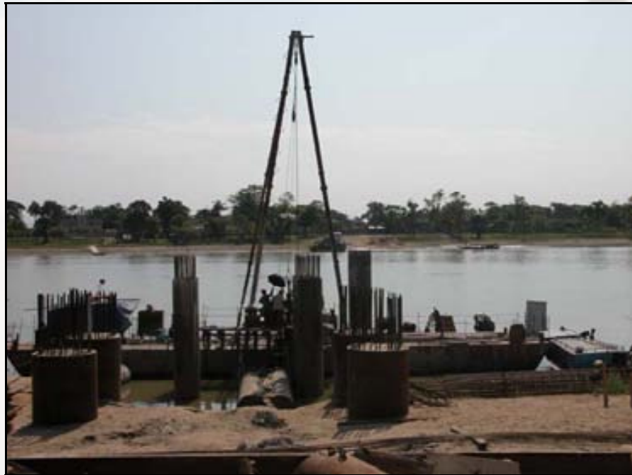
Construction of cast-in-situ piles with 1.4m diameter and 40m length for the jetty
