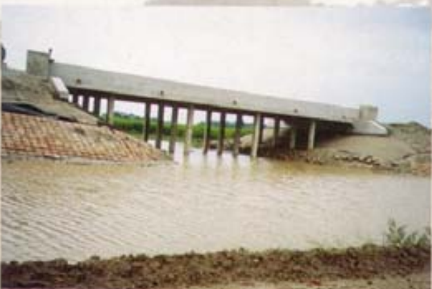
Slab Bridge (31 m) on 28.4 m Pre-cast Driven Pile at Ch : 2+645, Contract No. 3, JMB Project, Tangail
