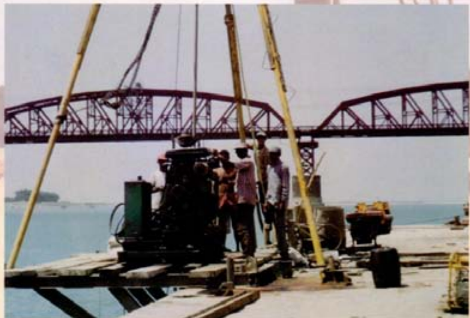
Exploratory Bore Holes by Rotary Drill Rig on River at Paksey Bridge Construction Project.
