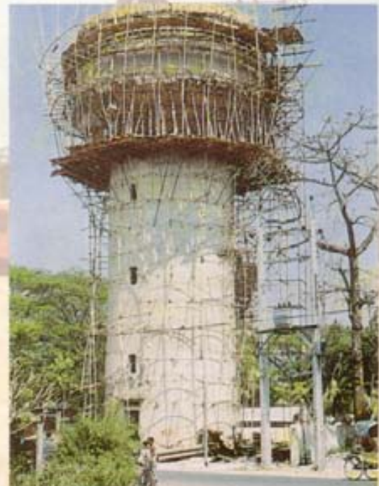
Construction of Top Dome
