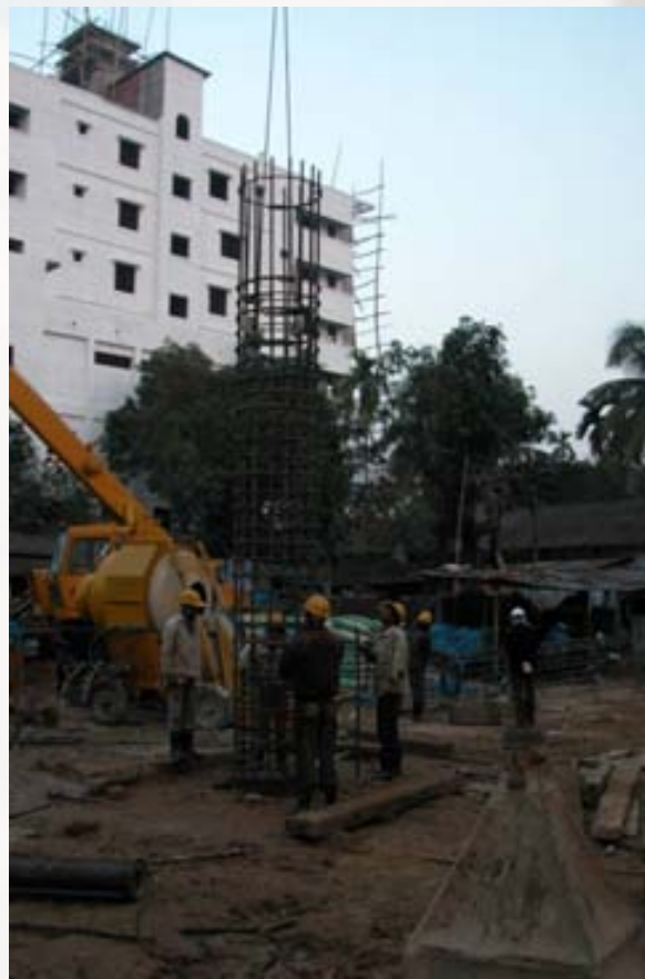
Lowering of Rebar Cage
