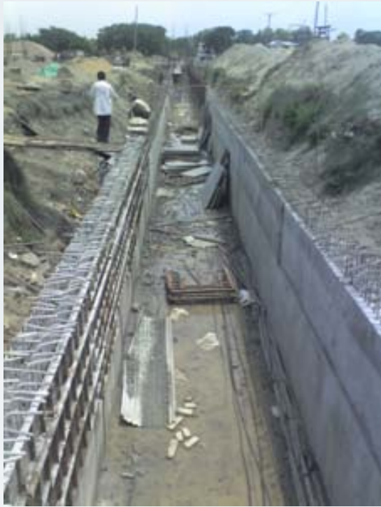
Construction of Tunnel for Conveyance System
