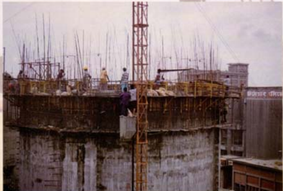
SLIP FORM in SILO Construction
