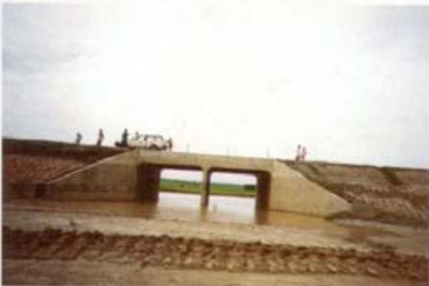
Double Cell Box Culvert at Ch : 4+400, Contract No. 4, JMB Project, Serajgonj
