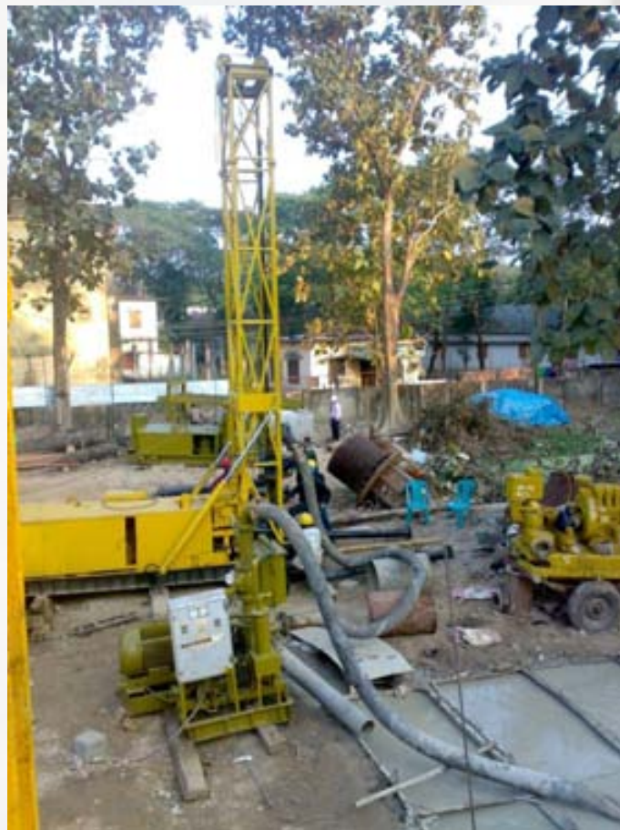
Reverse Circulation Drilling
