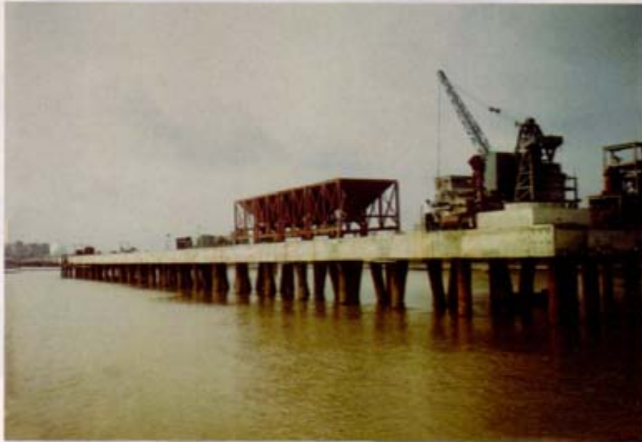
Completed Jetty for 10,000T DWT Vessel Berthing for Clinker unloading and Cement loading at Mongla Port
