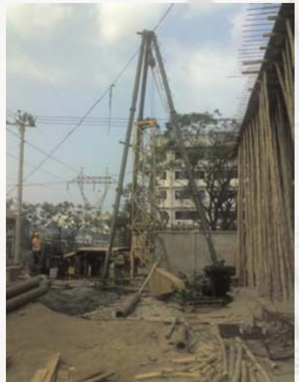
Drilling of 200m Deep Well
