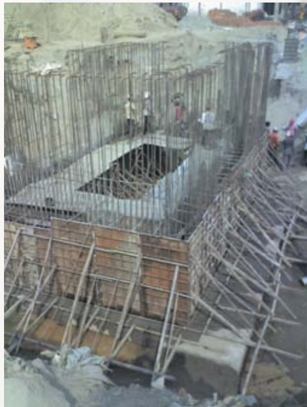
Construction of Tunnel 9m below Existing Ground
