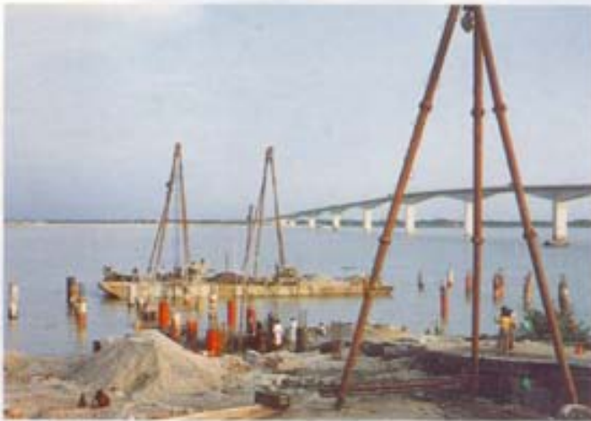
Onshore and Offshore Bored Cast-in-Situ R.C.C. Piles for Jetty, Length 52 m, Diameter 600 mm. Using Rotary Drilling Method.
