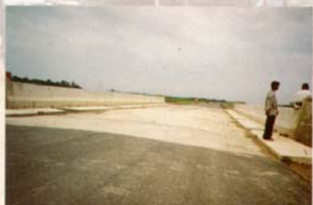
Slab Bridge (66 m) on 28.4 m Pre-cast Driven Pile at Ch : 1+725, Contract No. 4, JMB Project, Serajgonj
