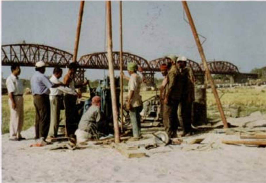
Exploratory Bore Holes by use of Rotary Drill Rig on Land at Paksey Bridge Construction Project.
