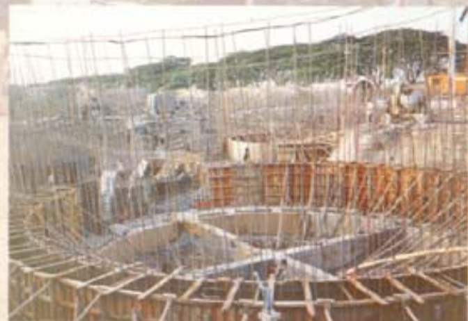
Construction of Clinker Silos
