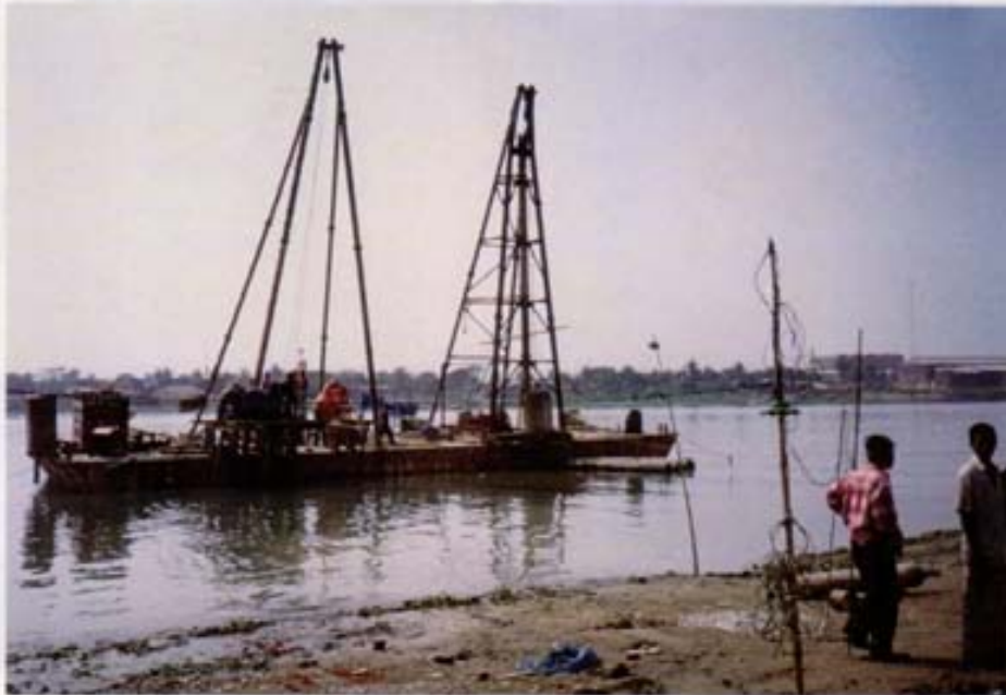
Off-shore Pile hole drilling by Rotary Rig for Bored Cast-in-Situ RCC pile for Jetty at Dhaka Grinding Plant Project of SCAN CEMENT
