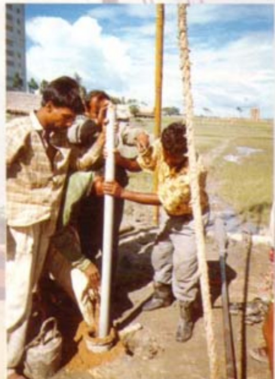
Lowering of Monitoring Well for Water Sampling
