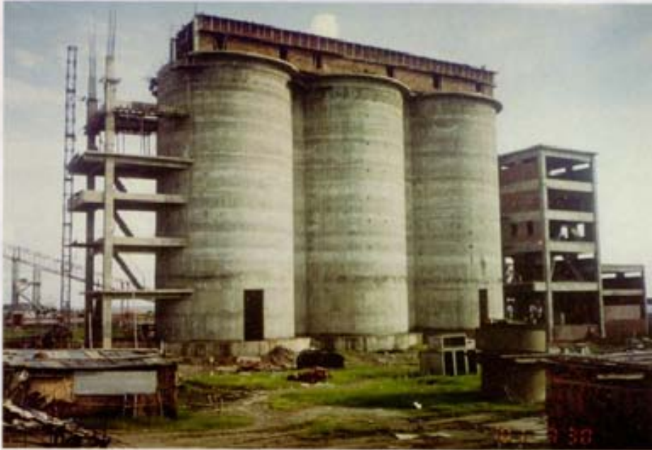
Completed 3 x 2000T Cement SILO using Slip Form Technique.
