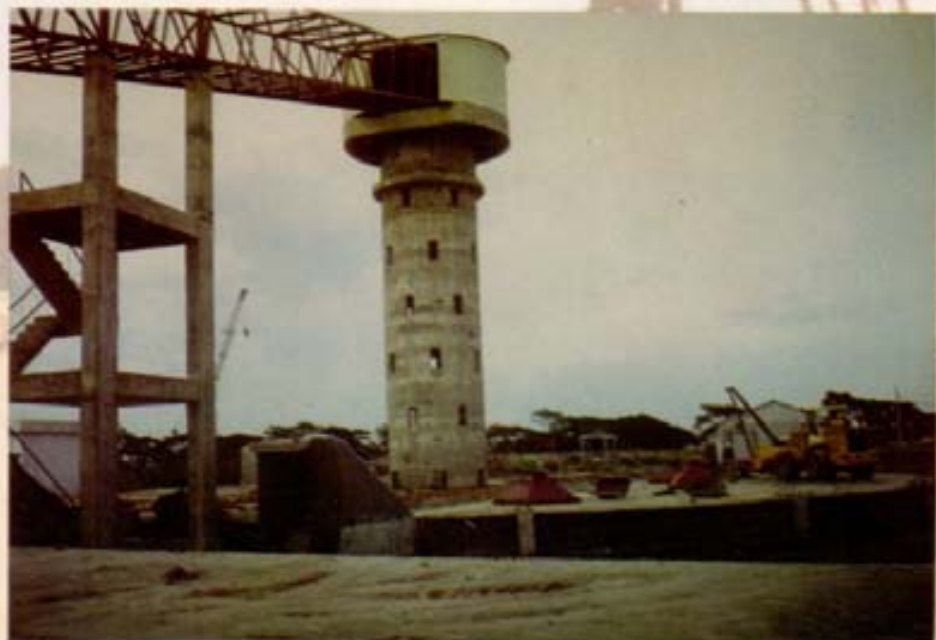
Clinker Storage at Mongla Port using Slip Form Technique
