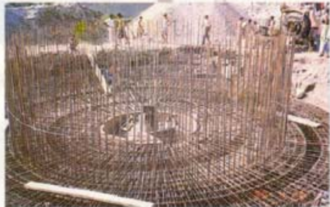
Construction of Pile Cap
