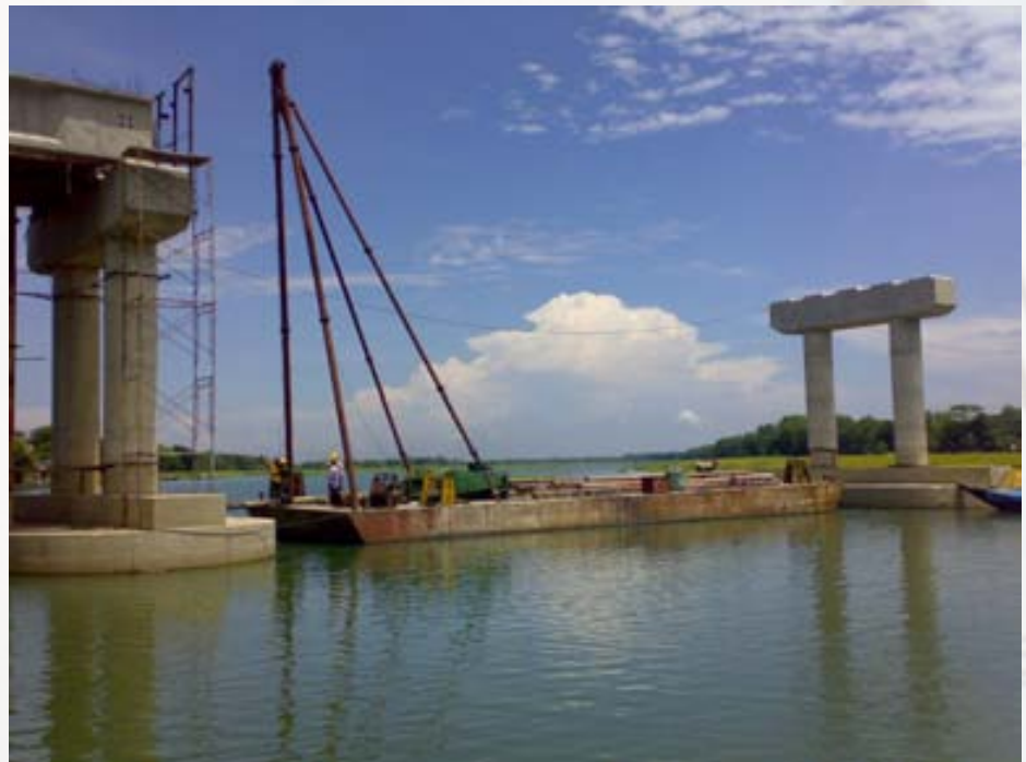
Construction of 1200mm diameter 38m long bored piles using rotary drilling method
