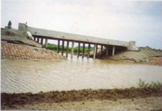
Slab Bridge (31m) on 28.4 metres Pre-cast Driven Piles at Ch : 3+335, Contract No. 3, JMB Project, Tangail
