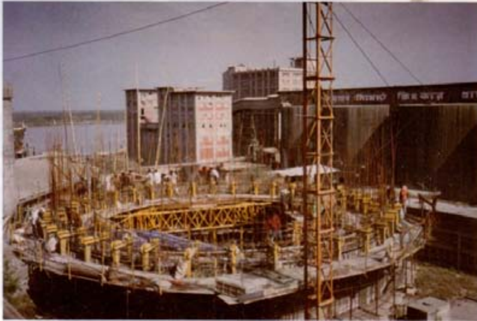
Cement SILO by SLIP FORM under construction
