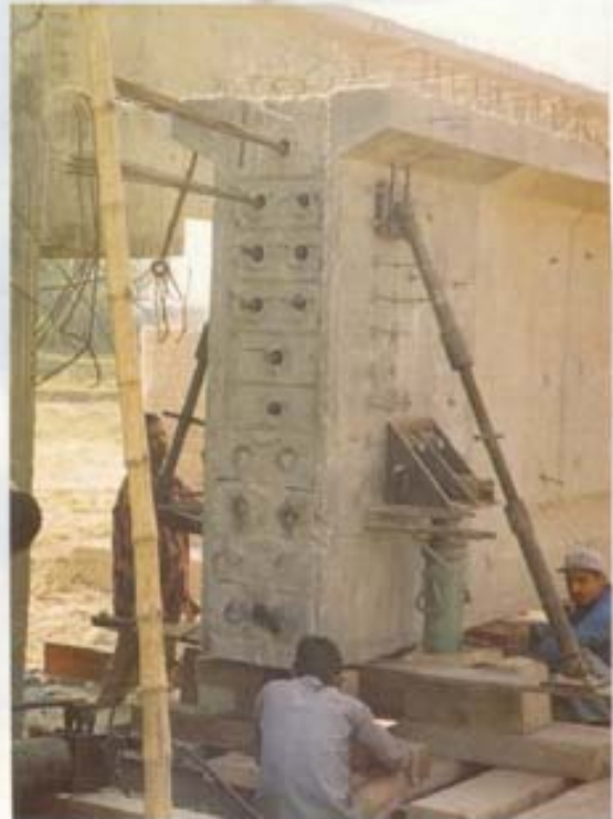
Lifting of PSC Girder from Casting Bed at Str: 20, Contract No. 9, RIP Project, Faridpur
