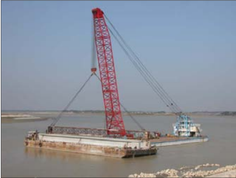
Lifting of 45m long PSC Girders from floating barge
