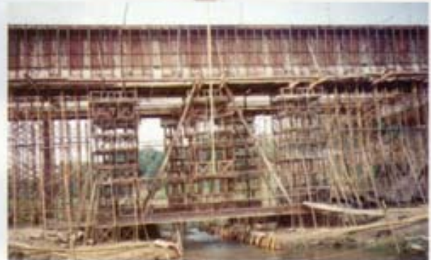
Scaffolding & Shuttering for concreting of Pre-stressed Girder in place at Str. No. 20, Contract No. 9, RIP, Faridpur
