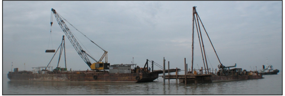
Installation of Offshore Fixed Platform
