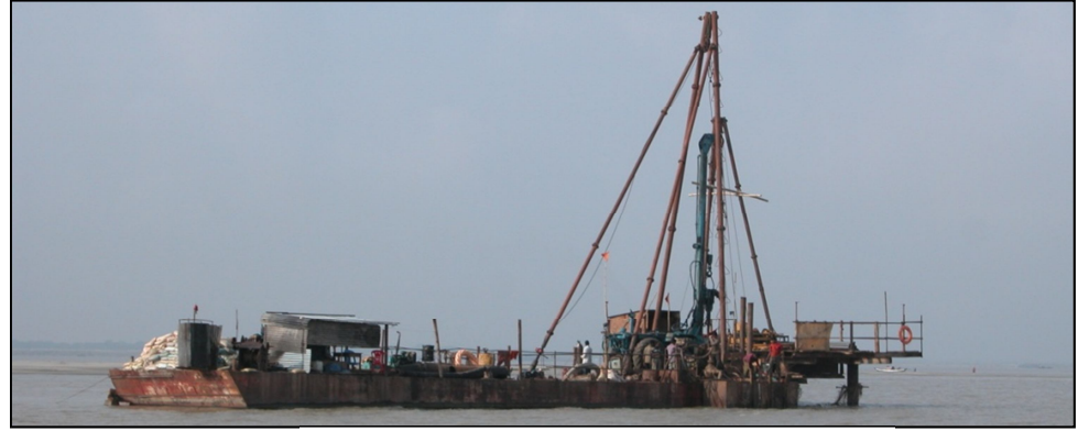
Drilling from Floating Platform
